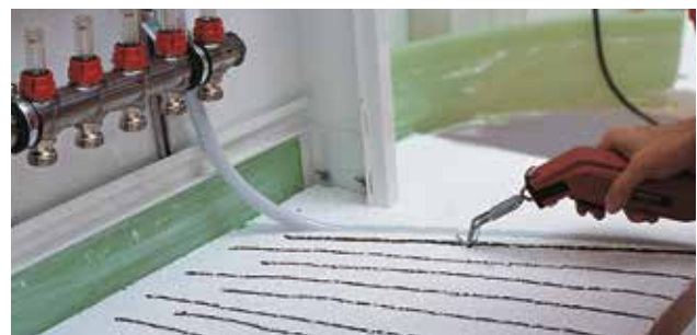
PRINETO heat-cutter for cutting individual pipe grooves.
