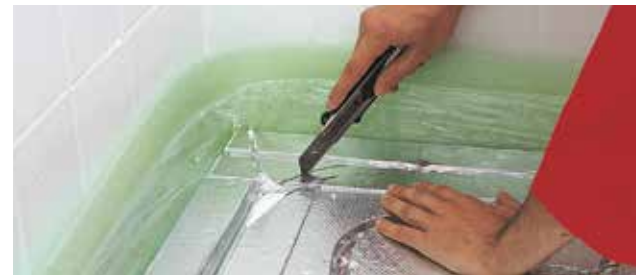
Connection of PRINETO grooved elements in corners.
